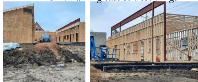
MARCH : framing east & west wings
