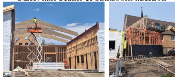
MAY: lam beams & bathroom addition
