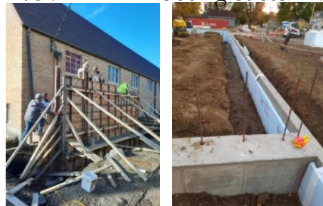
NOVEMBER: footing & stem walls
