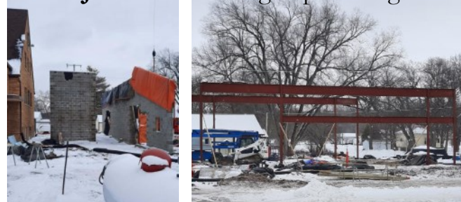
JANUARY: framing & plumbing
