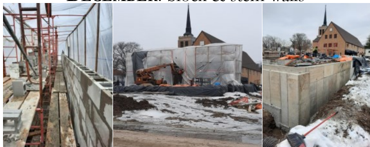
DECEMBER: block & stem walls
