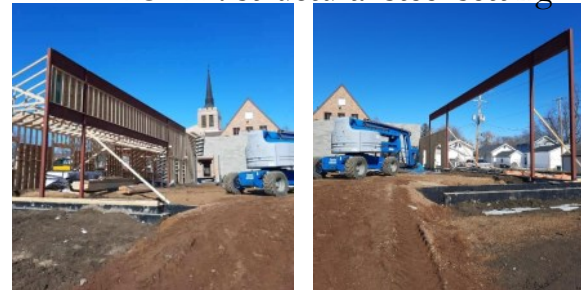
FEBRUARY: structural steel setting
